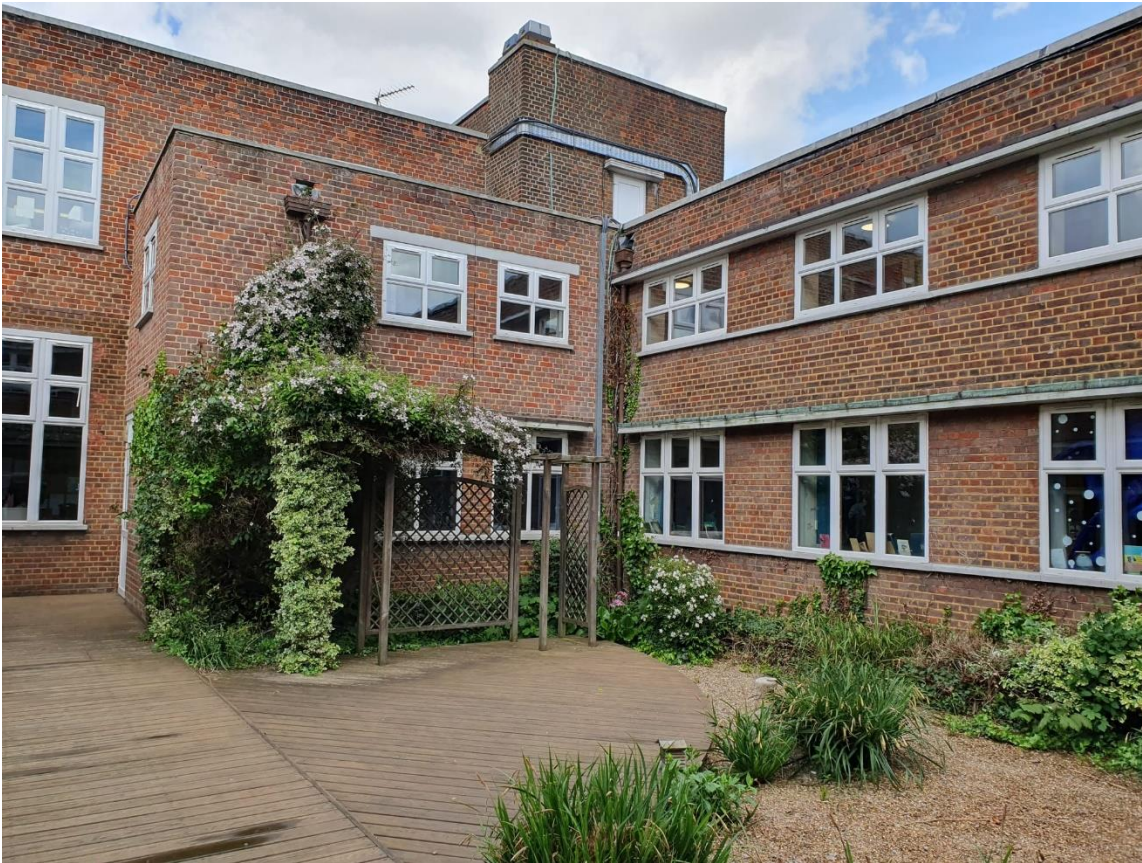
View of Courtyard and Protruding Element:
