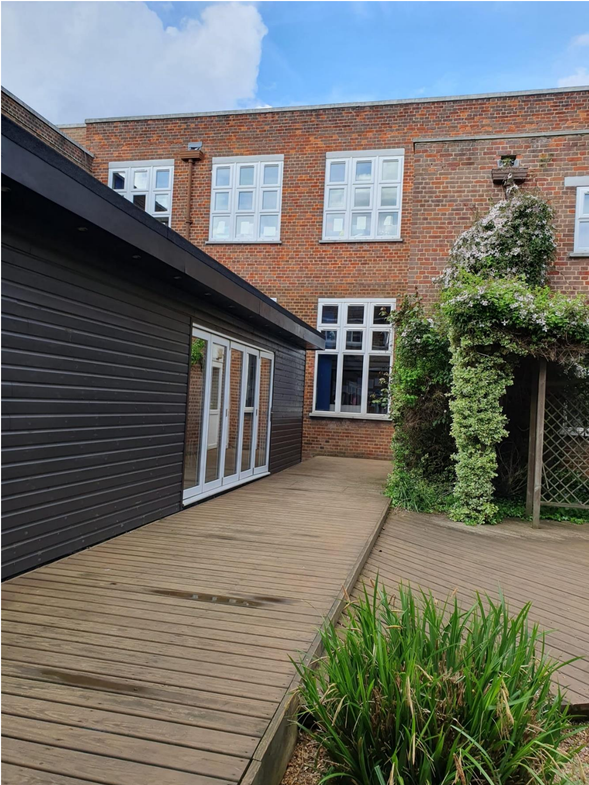
View of Courtyard and Existing Timber Outbuilding
