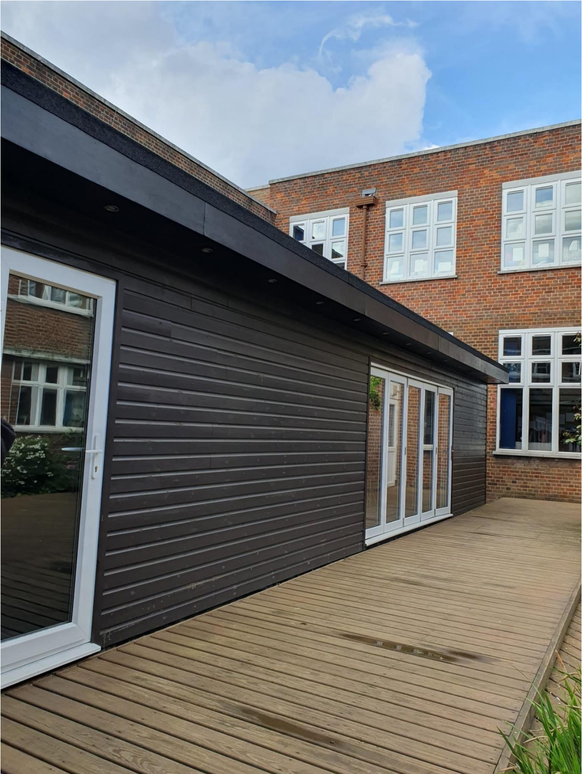
View of Timber Outbuilding:
