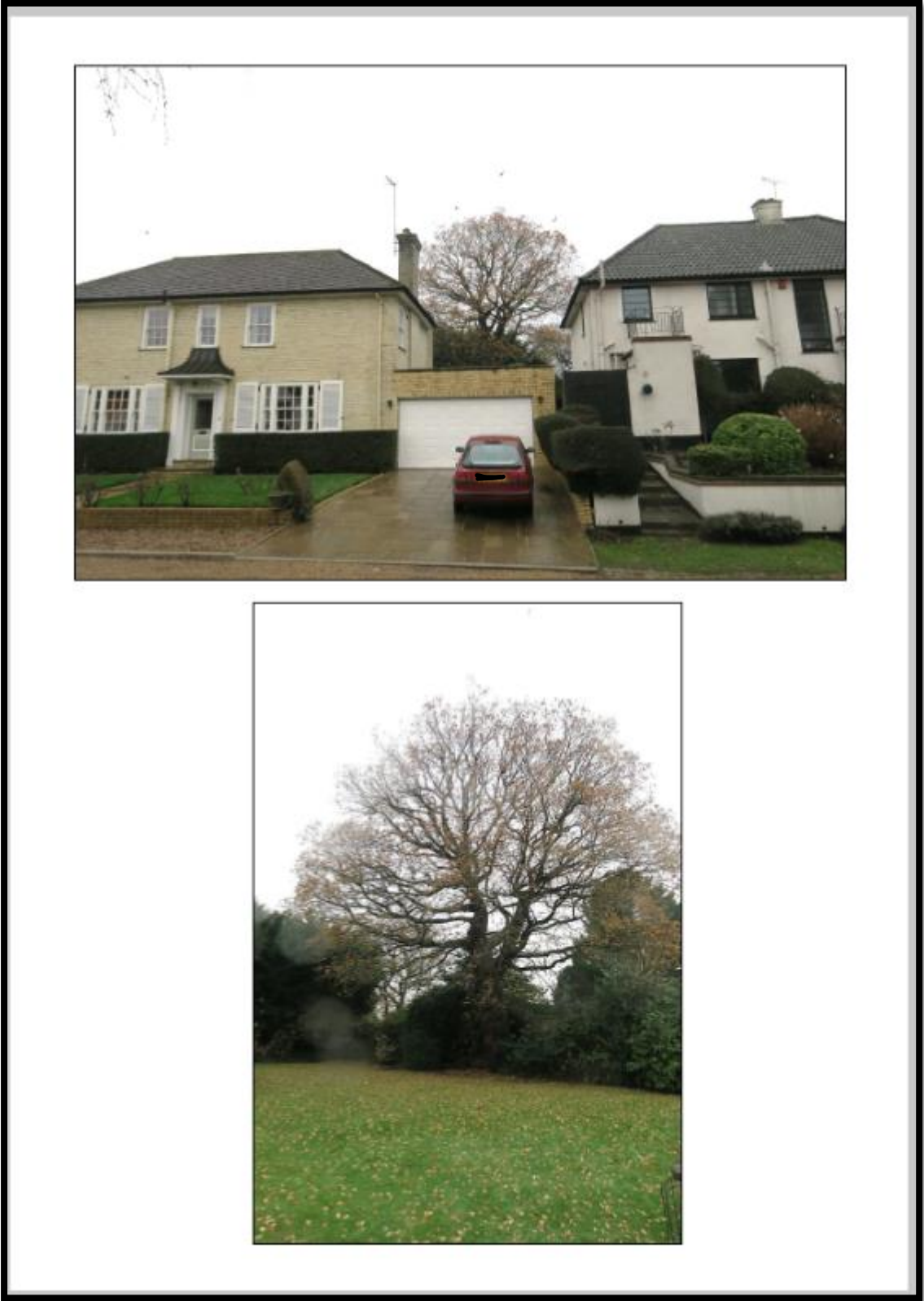
Top: T1 Oak viewed from East End Way Bottom: T1 Oak viewed from rear garden of Maribar
